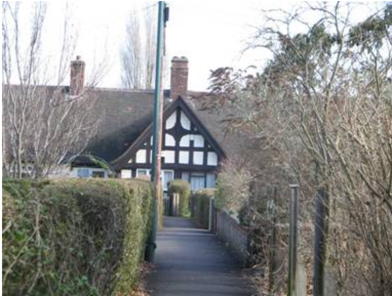
Photograph 4: Timber framed gables are common on the 1930s brick houses
