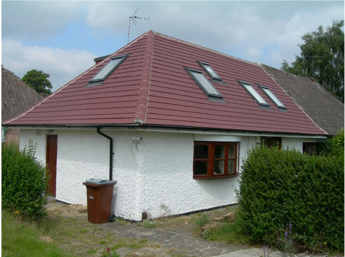
Photo 6: Altered Roof Claddings
