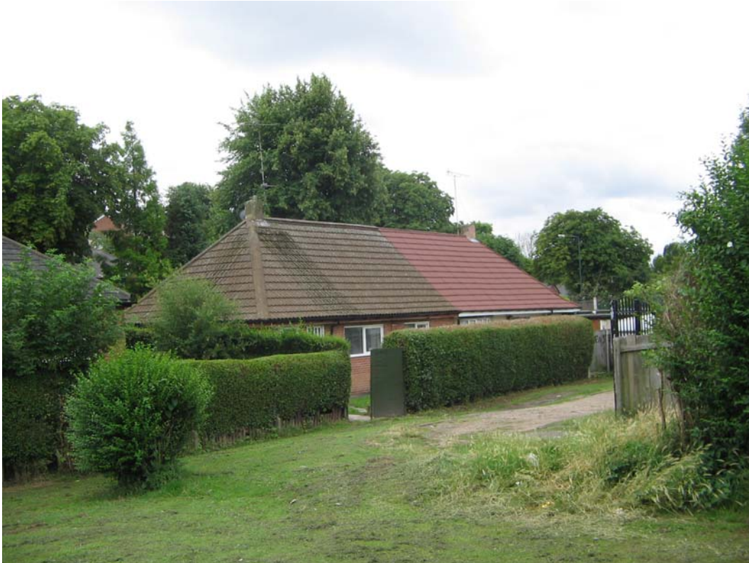
Photograph 1: The demonstration Crane Bungalows, The Wells Road
